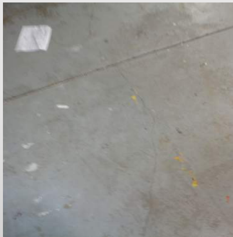
Concrete Cracking
