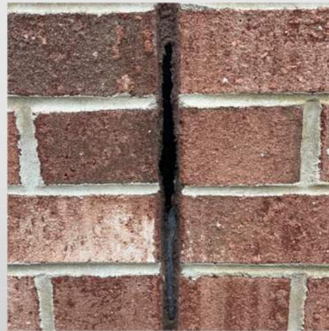
Windows, Doors, Frames & Caulking
