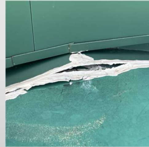
Wall Flashing, Coping Cap & Metal Panels
