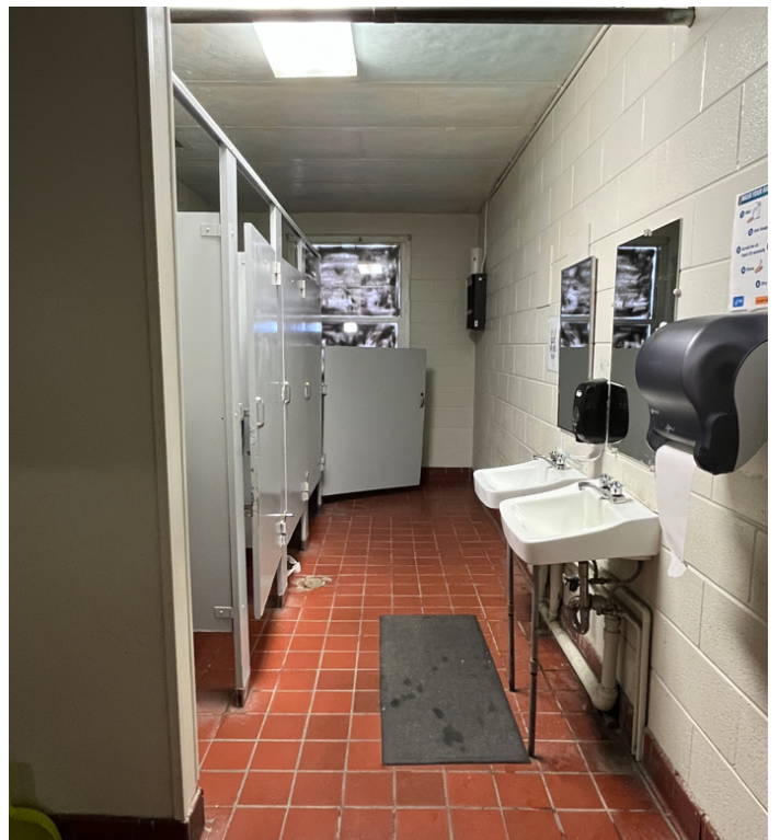
PHOTO AA.11 GROUP TOILET ROOM(S) - GRAB BARS, PATH OF TRAVEL, CLEARANCES & FIXTURES (ADAAG 309.4, 604.3, 604.5, 606.5 & 609.3)
