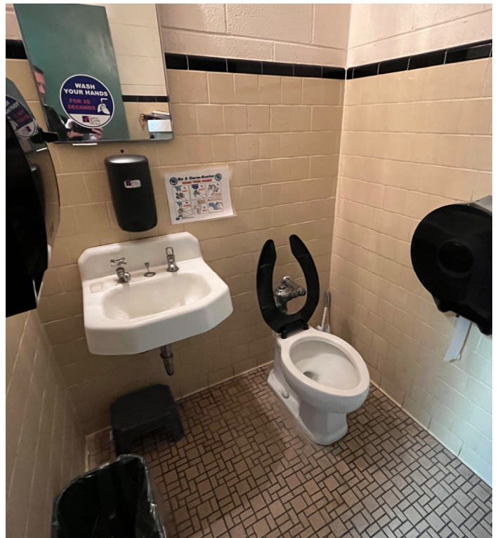
PHOTO AA.07 TOILET ROOM(S) - FIXTURE CLEARANCES, GRAB BAR SPACE & EXPOSED PIPES (ADAAG 604.3.1, 604.5, 606.5 & 609.3)
