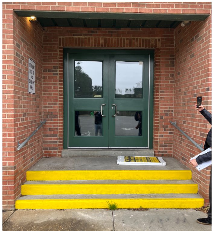
PHOTO AA.01 BUILDING ENTRANCE - ACCESSIBLE EGRESS AND HANDRAIL EXTENSIONS (ADAAG 402, 505.10.2, 505.10.3)
