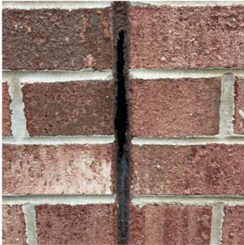
Windows, Doors, Frames & Caulking
