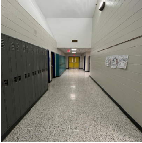
Finishes (Flooring, Walls & Ceilings)
